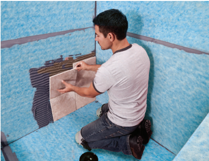
Waterproofing the shower base and walls ▶
